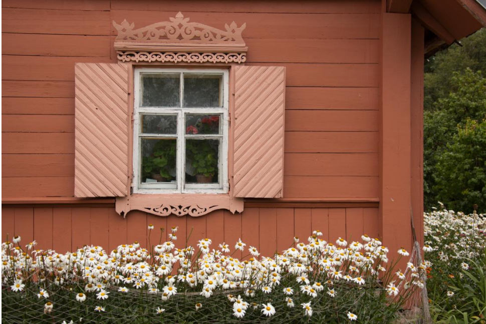
Photo: Māris Justs. Traditional window ornaments in Latgale. In scenic environment such facades are often replaced by a plastic covering which minimizes the visual charm of houses.
